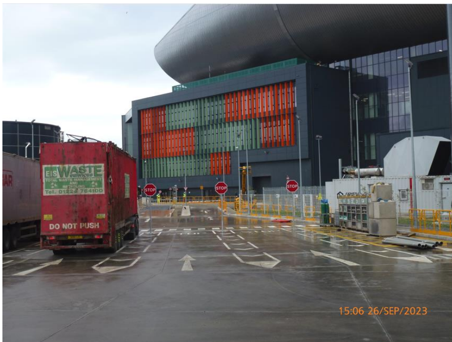
Staff parking area looking towards office block
