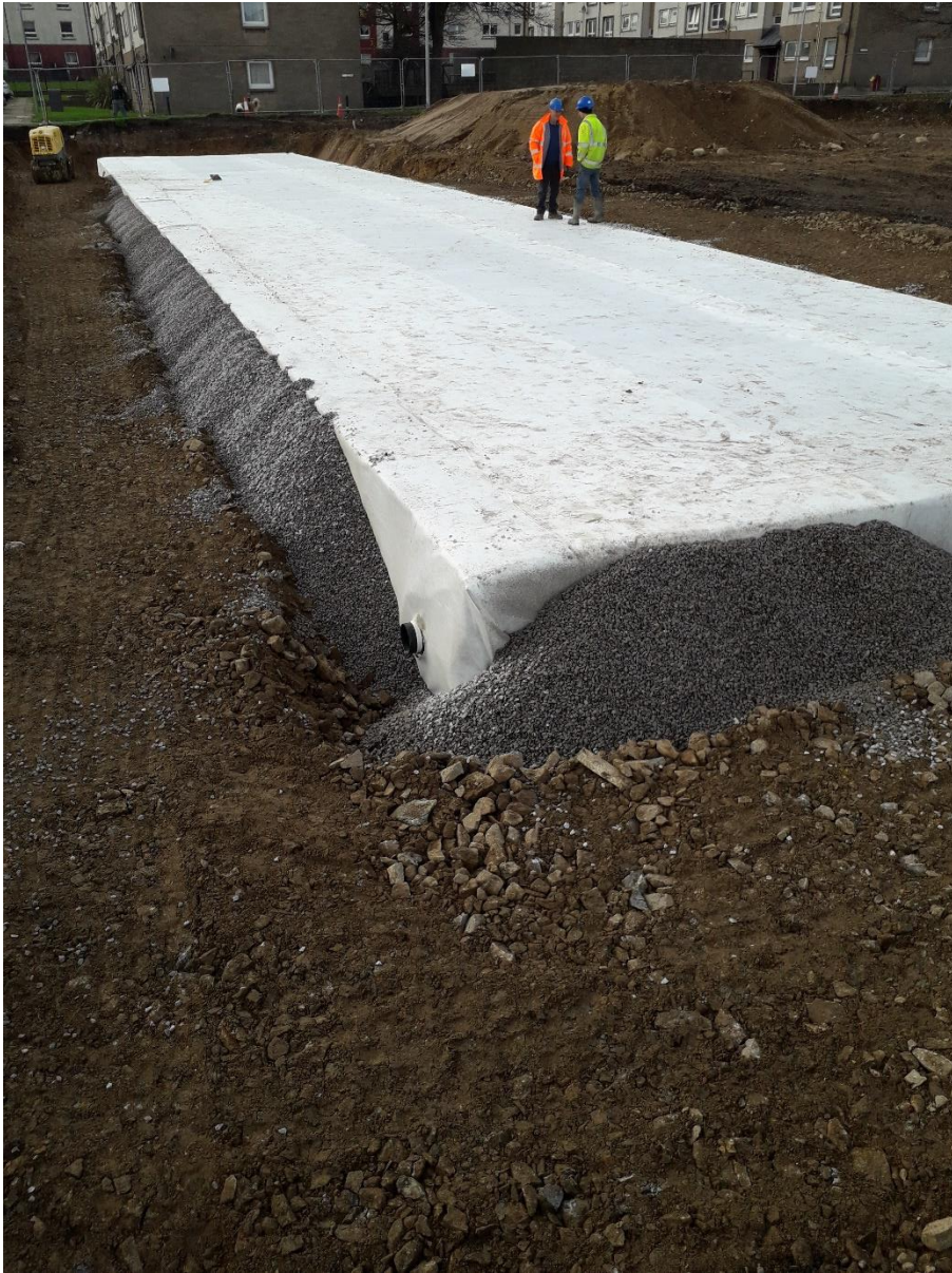
Attenuation tank installed
